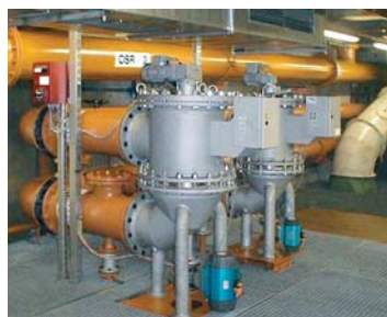
Cooling lubricant cleaning using automatic back-flushing filter RF3® for flow rates up to 50,000 l/min per filter.
