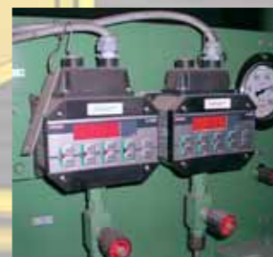
Pressure Switch EDS 1700 for wall mounting.
