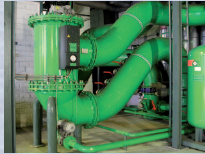
Automatic back-flushing filter AutoFilt RF3® (cooler protection)
