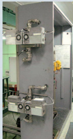
High pressure water filter RFH for the control of the water spherical valve
