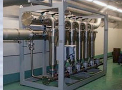
Automatic Twist Flow Strainer ATF® (for water pre-filtration)
