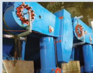
Servo motor (hydraulic cylinder on spherical / butterfly valve)
